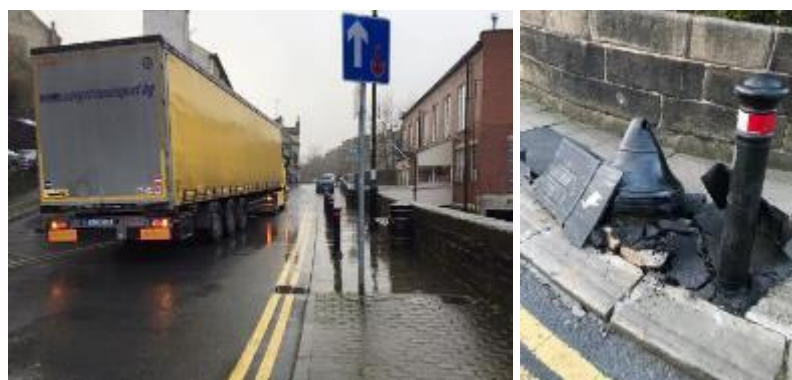
Figure 33 - Truck stuck on Hollowgate, Holmfirth & HGV damage to 'bell' protecting bridge on Hollowgate
